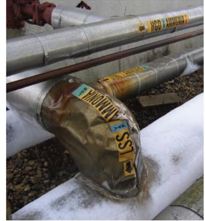
*Photo 4 (left): Corrosion to the pipe surface is not limited to the point of the insulation system failure. The piping down to the elbow and beyond also should be inspected. Photo 5 (above): The ever-present ice on the jacket of this pipe indicates possible failure of the insulation system.*
