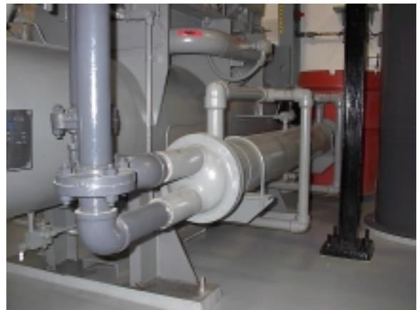
**Figure 1: Glycol fluid cooler (left) for screw compressor external glycol oil cooler (right).**
