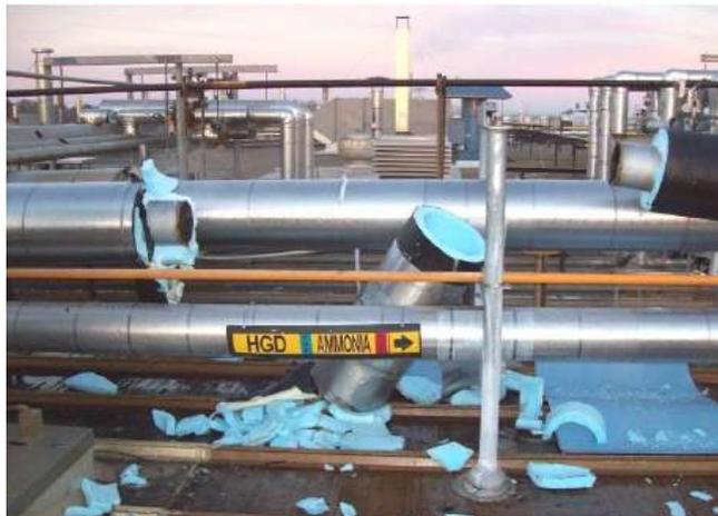
There are multiple issues with hot-gas defrosting evaporators that can exacerbate hydraulic shocking or hammering:
